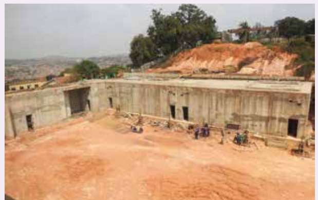
New Radiotherapy bunkers underconstruction
